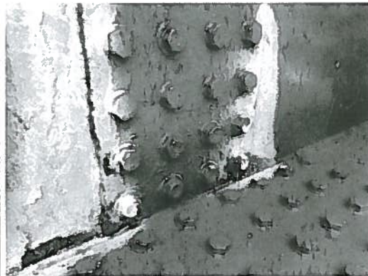
12. Trolley girder lower web plates at bolted splice beneath machinery house are corroded through.
