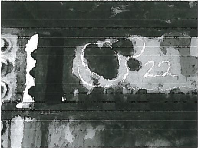
10. West landside trolley girder to sill beam. Gusset – Severe corrosion
