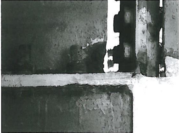
10. West landside trolley girder to sill beam. Gusset – Severe corrosion
