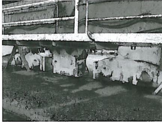
11. Boom bolted splice plates at underside of top flanges (typical left and right) are corroded to approximately 50% of original thickness.
