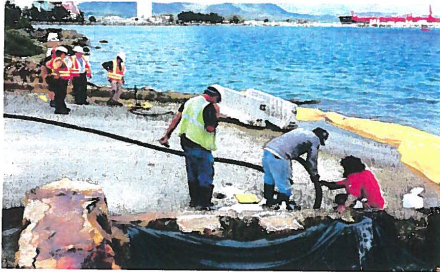
Trident Cross working on infusing concrete into Seaplane Ramp.
