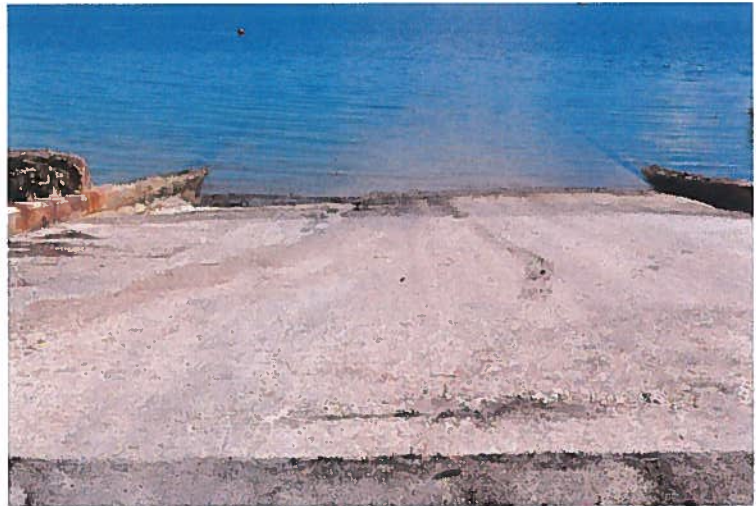
Seaplane Ramp repair completed.
