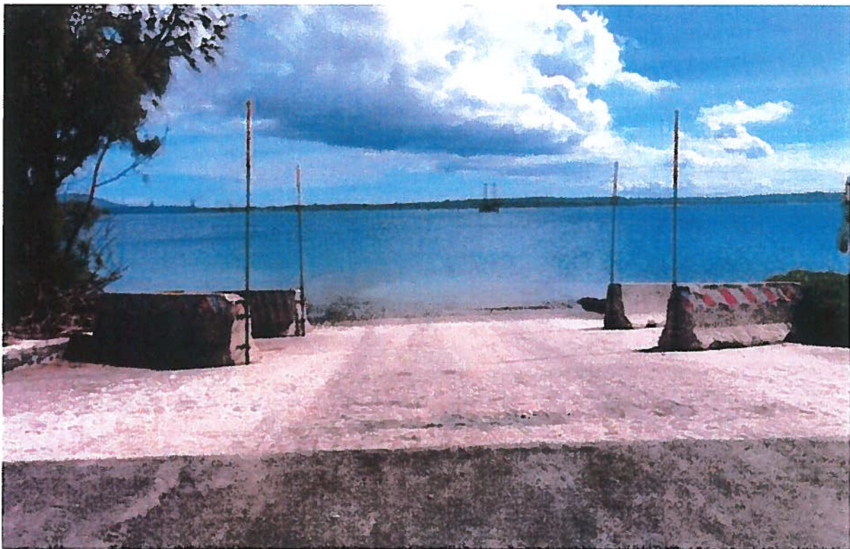
Jersey Barriers installed to ensure that boats travel at center of the ramp. Boating activities include the “Duck Boat” operation, recreational boats or jet skis.
