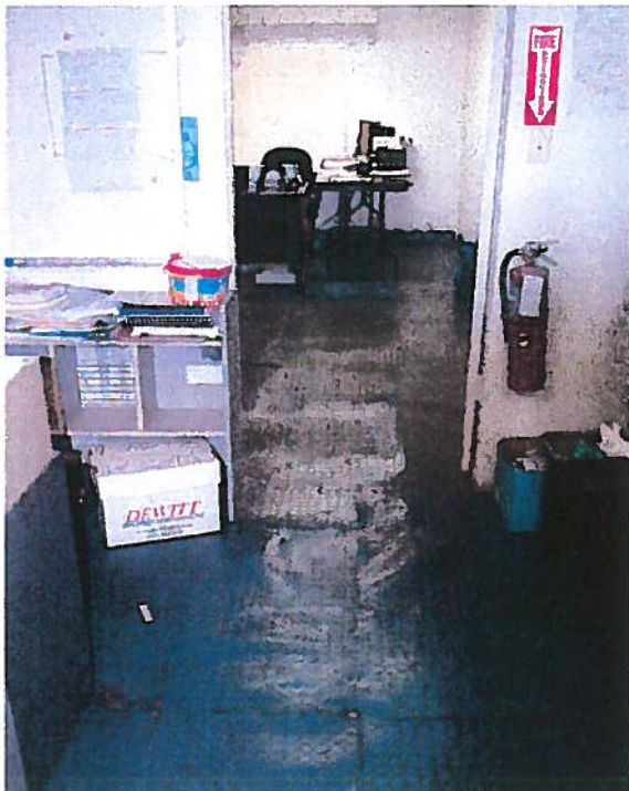
The unevenness of the floor in the Safety Office is due to termite infestation creating a tripping and safety hazard.
