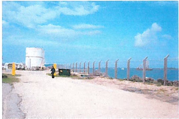
Completion of F1, F3 Container Yard South Side Security Fencing Project.
