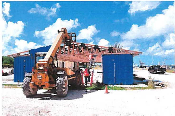
Demolition in Progress on EA Field Office building.
