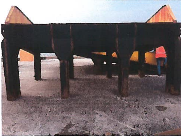
Damage at F3 pier pavement caused by the ramps metal plate scraping back and forth during the aggregate operation of loading gravel.
