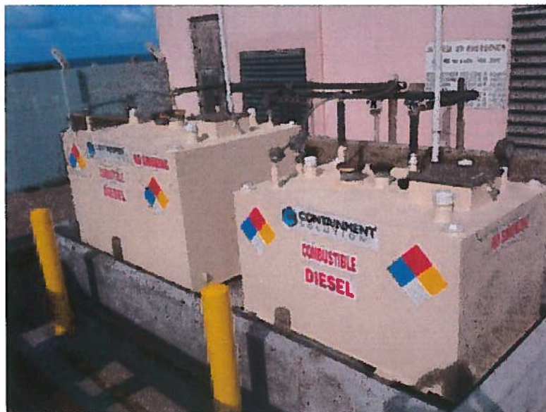
Installed External Day Tanks (1,000 and 500 gal.) for LC-4 Generators.
