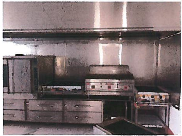
Newly installed restaurant equipment.
