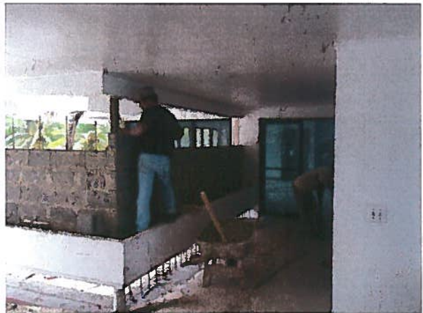
Front entrance renovation in progress.
