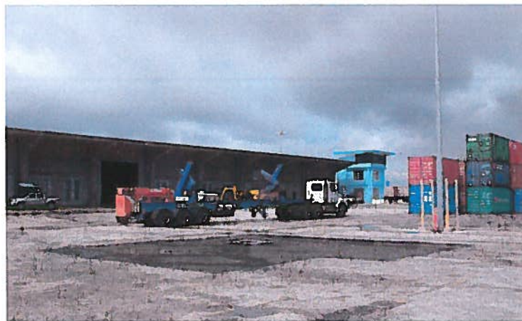
Oil Water Separator 3
