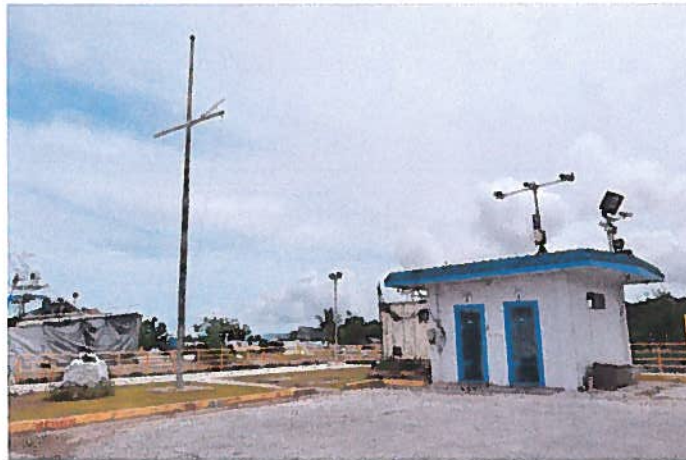
Potential site for GFD Rescue Unit.
