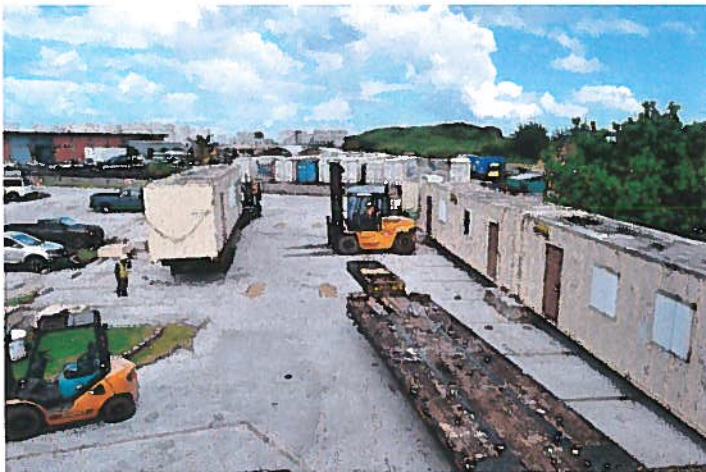
Removal of Temporary Container Office Space.
