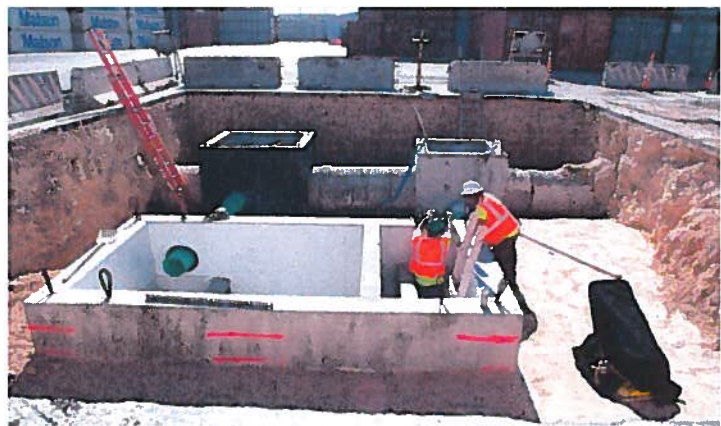
Construction work being performed on Oil Water Separator 8
