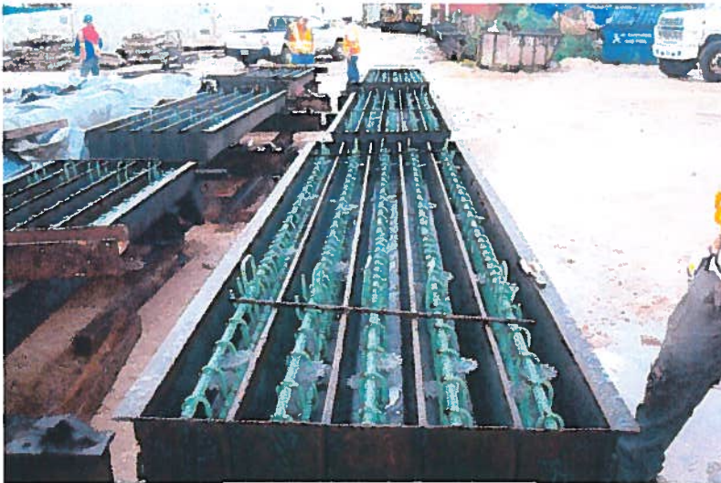
Security Fencing Project ongoing.
