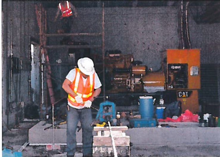
Construction work being performed to install Load Center 4 Generator
