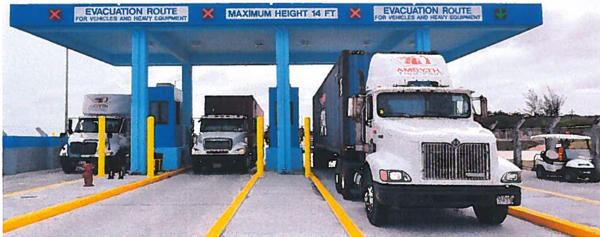
New Terminal Gate Complex
