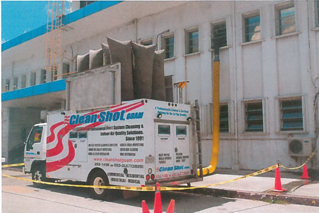
June 30, 2015: Clean Shot company performing work on the air-con ducts.
